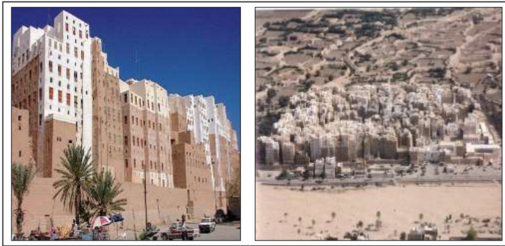
Figure 2: Shibami houses (mid and high-rise buildings)
